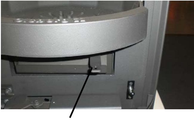
Operating lever for the fire grate
