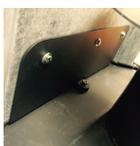
**7:** Place the stone against the metal plate with the threaded holes in line with the prepared holes, and fix it in place with a 10 mm socket spanner.
