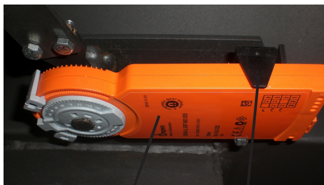
Servo motor Motor retaining clip
